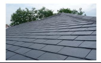
Estillo 15 is available in two selection grades – Prime and Premium. The Prime grade is the best selection that the quarry can produce, which will give a cleaner crisper roof line. The Premium grade has more variation in thickness and flatness and requires more grading prior to fixing, this will give finished roof with a little more character.
