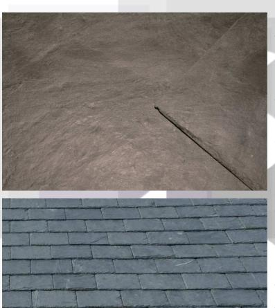
Samaca Q53 is a dark blue grey slate produced in the Los Molinos region of Northern Spain. The slate has a good natural texture giving the appearance of a domestically quarried slate to the finished roof. The duller texture of the slate is in contrast to many imported slates which can have a very noticeable sheen on the roof.
